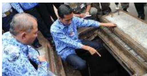
Figure 1 Branding Jokowi, an official who is willing to enter a culvert (December 16, 2012)
